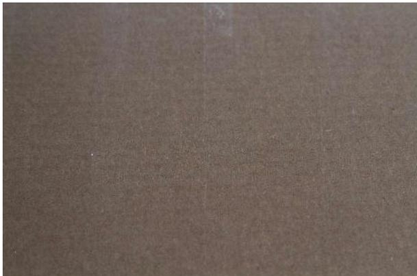
Figure 8: Application on a work surface: stripes are barely visible and it is difficult to monitor the progress of work.
