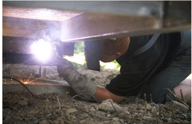
Figure 7: ... and welded onto the turntable, which had been put into an exactly horizontal position.
