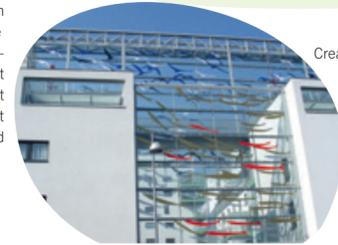
Creative designs on noise barriers increase the design value of a structure, but must be tested for their effectiveness according to ONR 191040 'Bird Protection Glass'.
